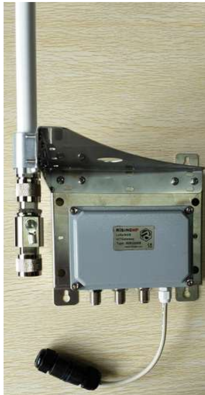
(3) surge protector fixed
